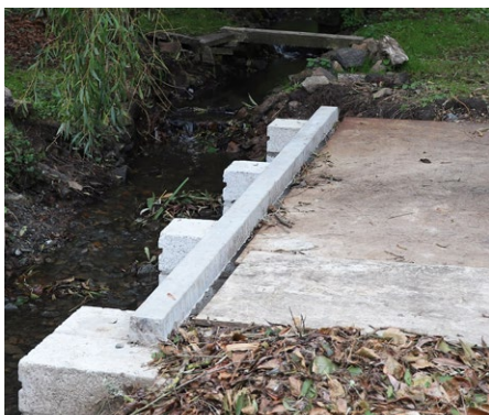
L-R: Before and After: following the collapse of the old stone culvert at Moulin de Quanteraine, the Trust has successfully replaced it with a new 450mm land drainage pipe and inlet structure.
